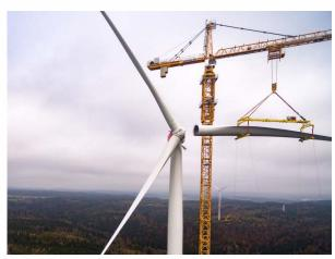
Figure 4: Attaching the leaves. Foto: © Max Bögl Wind AG, photographer: Holger Hessenthaler.
