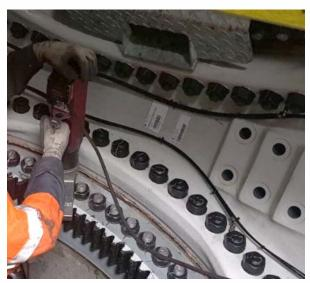
Figure 5: Bolting connections under confined conditions in the rotor housing.
