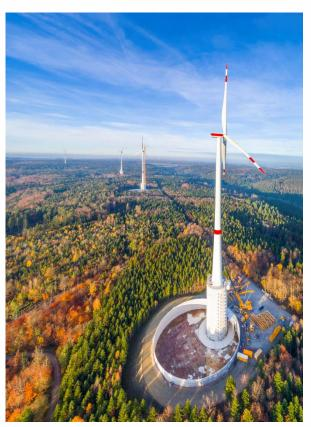
Figure 1: The natural battery storage in Gaildorf. Foto: © Max Bögl Wind AG, photographer: Reinhard Mederer.
